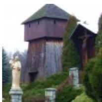
Next to the church a free standing belfry overlooks the area. This building was erected probably in the 17th century. The tower possesses post and beam construction with the walls narrowing towards the top. It is crowned with an overhang ice breaking pier covered with a pyramidal, shingle roof.
